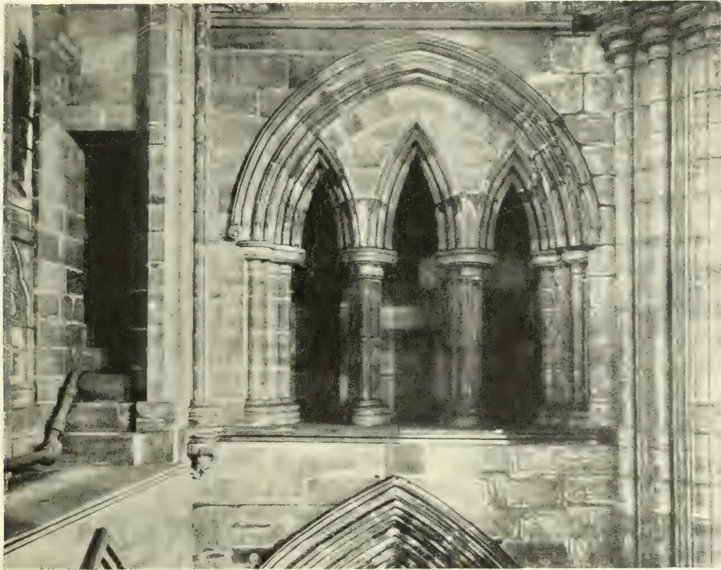
Triforium, East side of North Transept.
